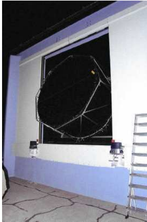
Figure 3.6: Picture of a drum mounted on the outside of the FD building for calibration.
