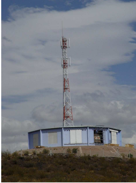
Figure 3.4: The Los Leones fluorescence detector building as seen from a point below and in front. The hatch coverings are motorized, opening during dark night periods to observe air fluorescence. Each hatch is for a single telescope.
