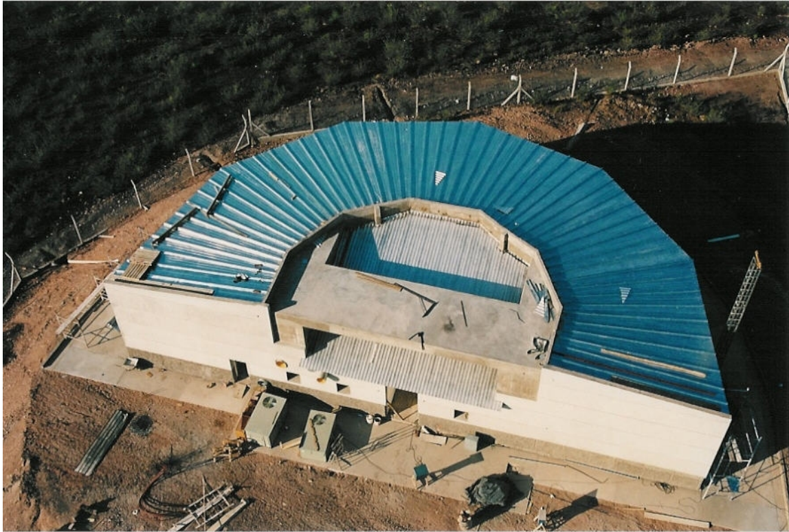
Figure 12: One of four FD stations on the periphery of the SD array. The FD station contains six mirrors that reflect fluorescence from the excited atmospheric nitrogen on an array of 440 PMTs.
